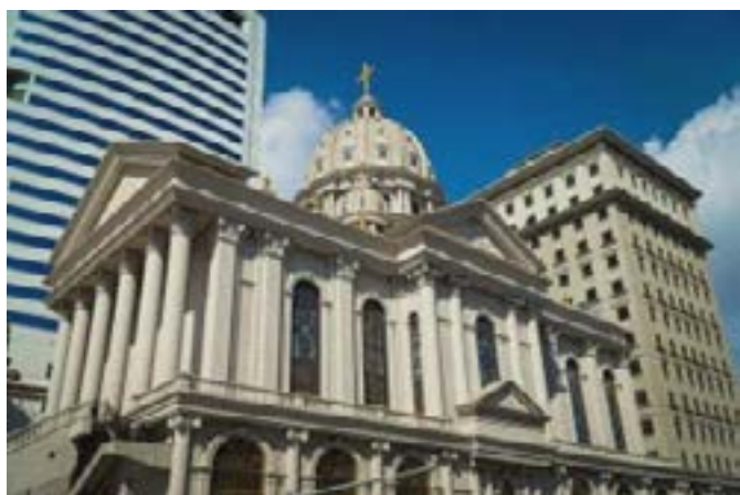
The Sacred Heart of Jesus Church in Kunming before its demolition in October 2021. Source: 163.com.
