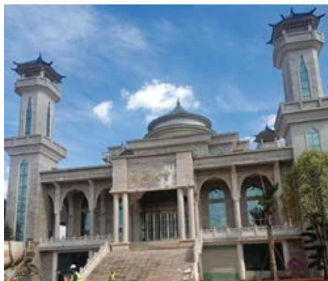
Tianxin Mosque, after the renovation. Source: CSW.
